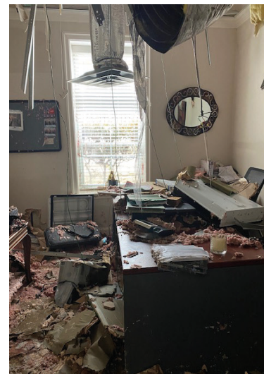
(Above) Water rushes out a door at the Dallas BA headquarters after hours of flooding. (Below) A burst sprinkler pipe resulted in collapsed ceilings and significant water damage.
