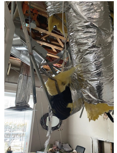
(Above) Water rushes out a door at the Dallas BA headquarters after hours of flooding. (Below) A burst sprinkler pipe resulted in collapsed ceilings and significant water damage.
